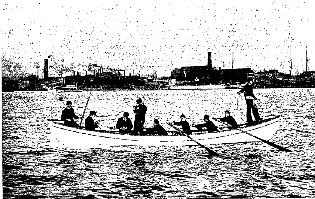
FIGURE 58.—Sounding with a handlead and line from a whaleboat in a survey of Baltimore Harbor on November 7, 1900.
