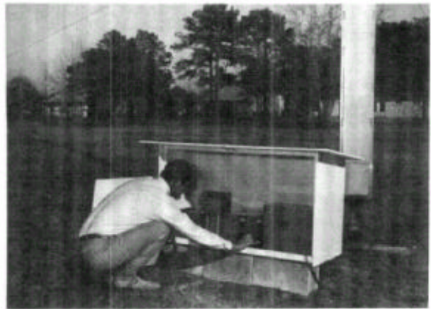
FIGURE AC-4. - Raydist shore station installation, (courtesy of Teledyne Hastings-Raydist, Hampton, Virginia)
