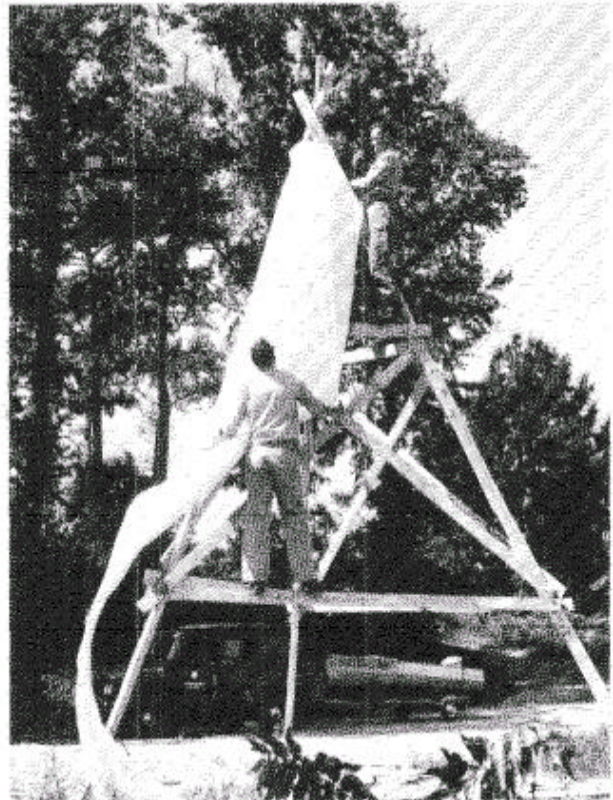
FIGURE 3 - 5. Construction of a large tripod signal
