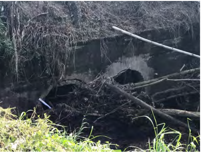
Figure 9. Examples of typical road crossing structures (Left: bridge; Right: round culvert). When structures are not properly designed, they disrupt river connectivity affecting the movement of migratory aquatic fauna (Photos: B. Yoshioka, USFWS, retired (left) and A. Galindo, USFWS (right)).
